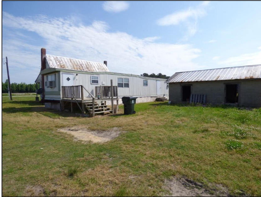
Photo 54: Mobile Home, Southwest Oblique.
