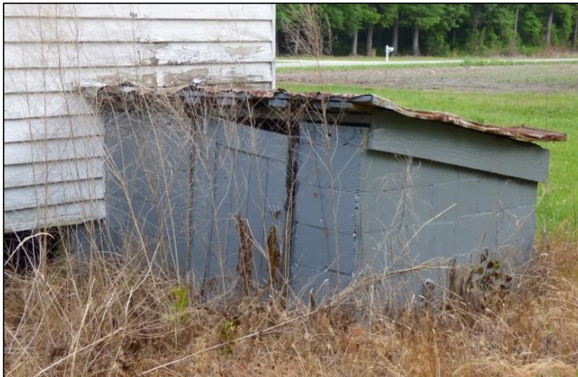
Photo 126: Cistern, Southwest Oblique.
