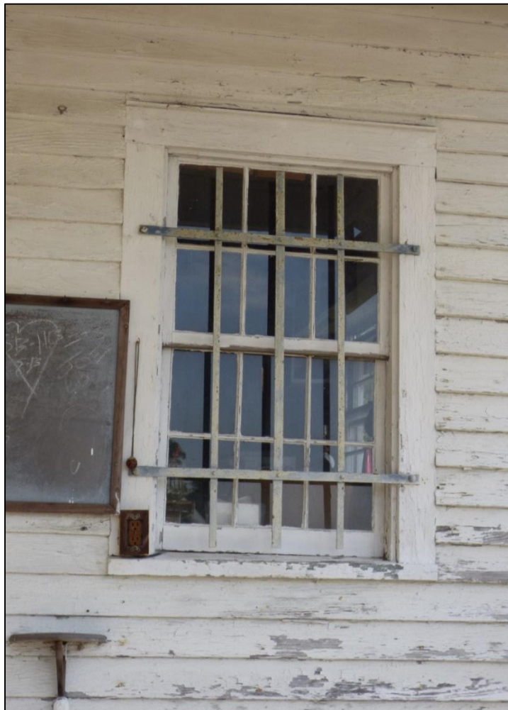
Photo 4: Window Detail on the Store, Looking Northwest.
