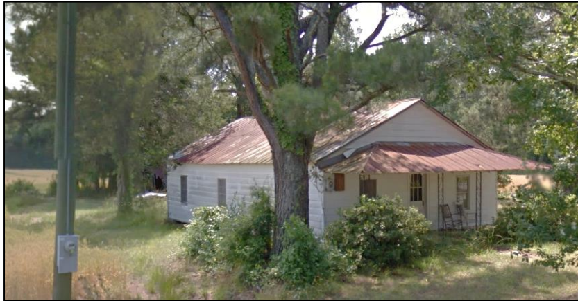
Photo 132: House at 3000 block of Leggett Mill Road (Google Street View 2015).
