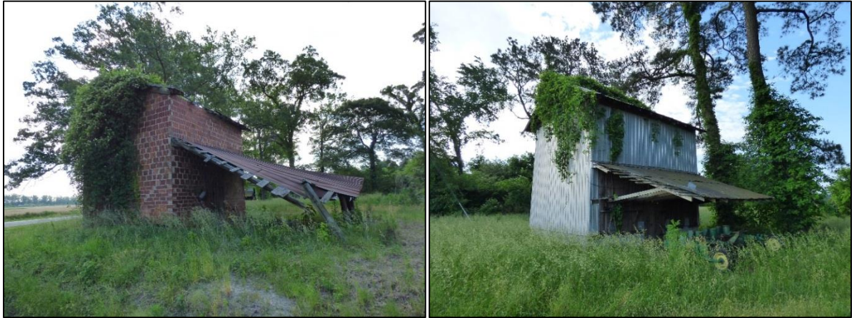
Photo 17: Clay-Block, Flue-Cured Tobacco Barn, West Oblique (Left) and a Frame, Flue-Cured Tobacco Barn, North Oblique (Right).
