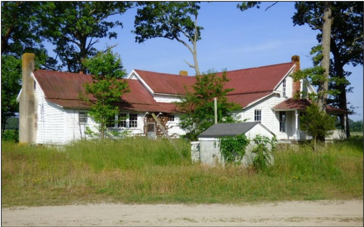
Photo 15: Dwelling and Additions, East Oblique.
