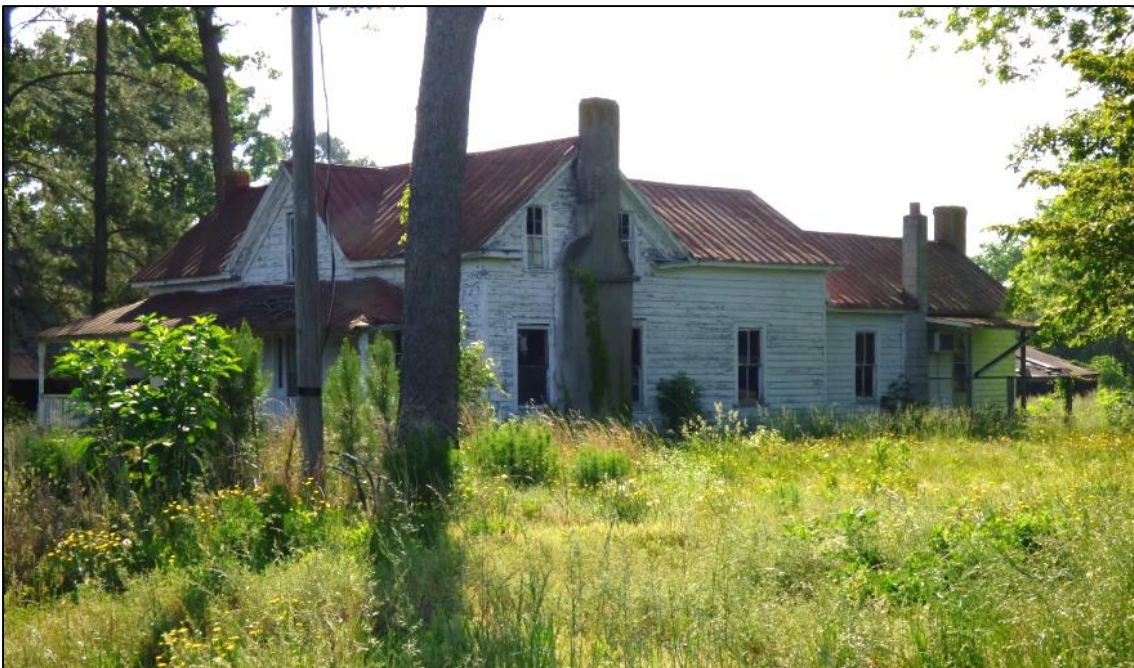
Photo 14: Dwelling and Additions, West Oblique.
