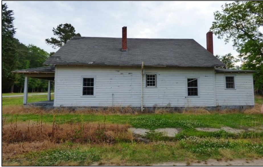
Photo 123: C.M. Wynn House, West Elevation.
