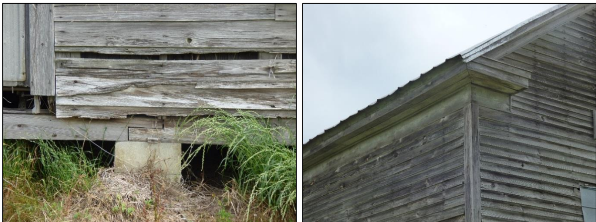
Photo 92: Primary Resource Detail of Foundation (Left); Detail of Roof Eave (Right).
