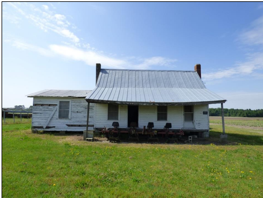
Photo 49: Façade (North Elevation) of the Alexander Mobley House.
