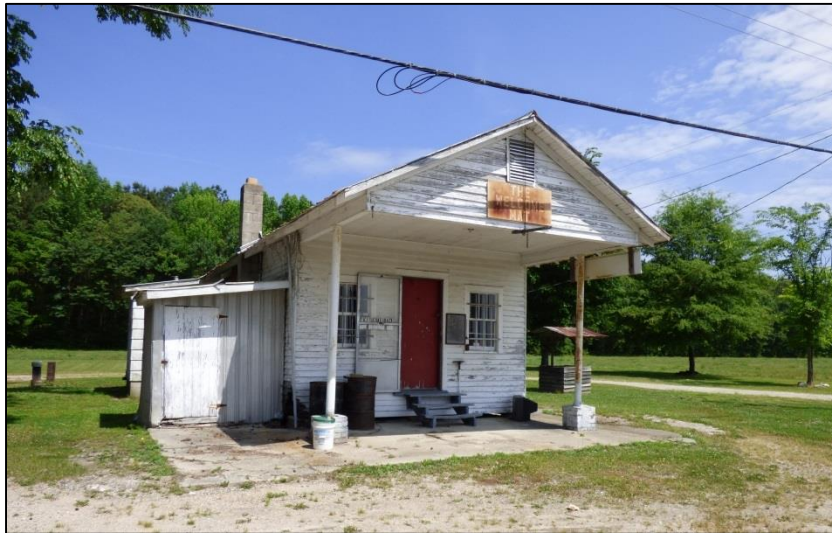
Photo 2: Store, Southeast Elevation.
