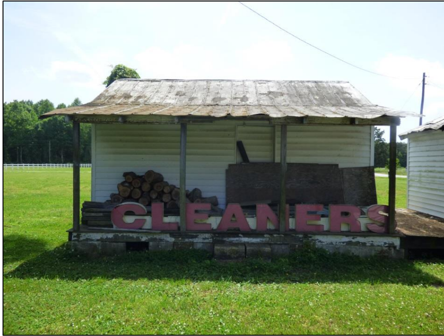
Photo 115: Detached Kitchen, Northeast Elevation.
