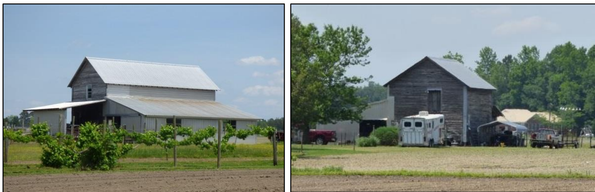
Photo 101: Northwest (Left) and Southeast (Right) Obliques of the Barn.
