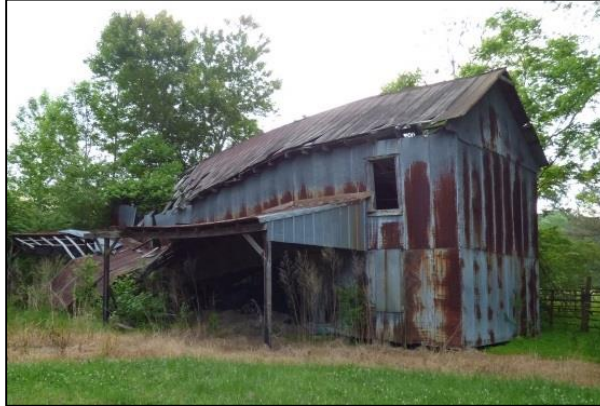
Photo 129: Barn, Northwest Oblique.
