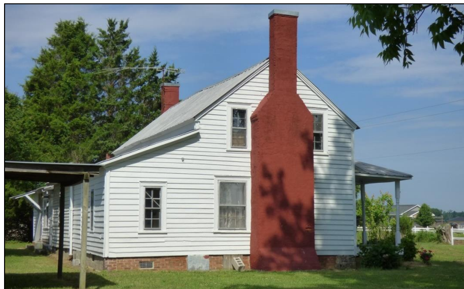
Photo 61: Southeast Oblique, Showing the Rear Shed-Roof Addition.
