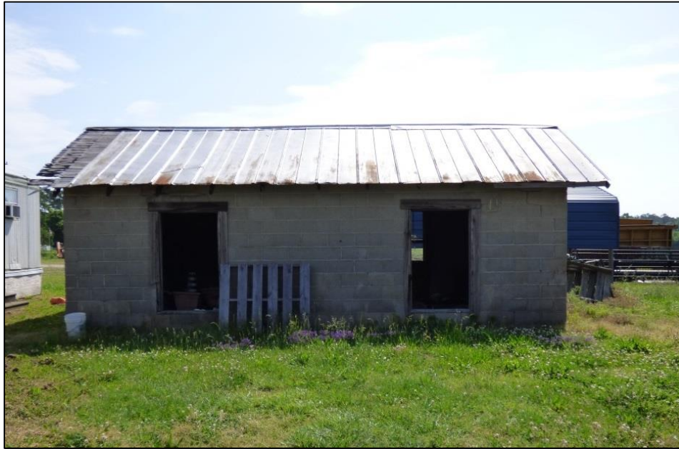
Photo 51: Concrete-Block Outbuilding, West Elevation.
