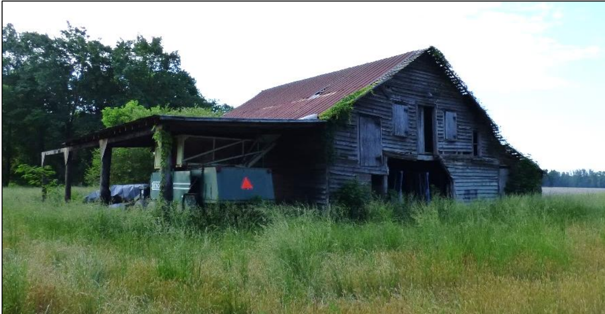
Photo 18: Frame Multi-purpose Barn, North Oblique.
