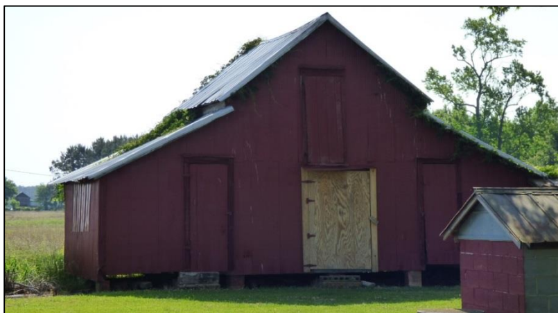
Photo 66: Packhouse, West Elevation.
