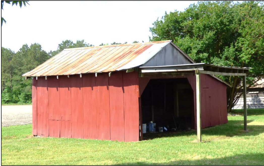
Photo 63: Garage, Northeast Oblique.
