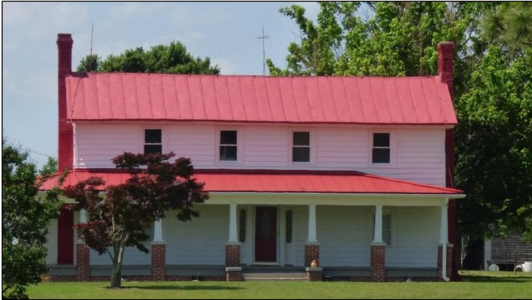
Photo 98: South Elevation of the Primary Dwelling.
