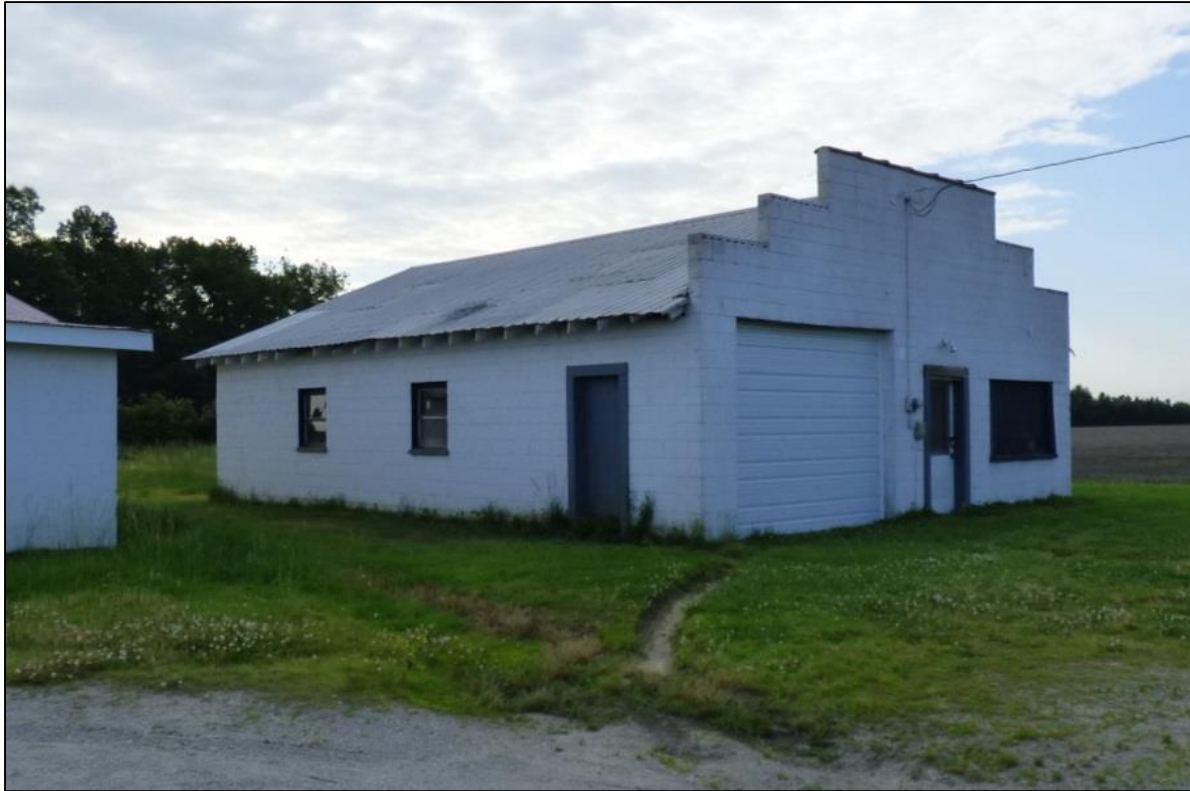
Photo 87: Garage on Leggett Mill Road, Northwest Oblique.
