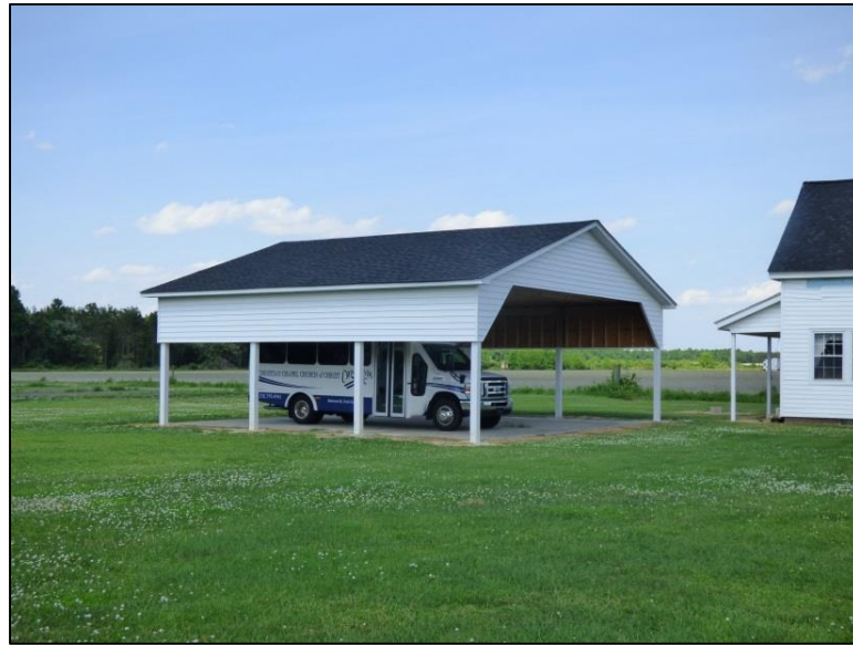
Photo 77: Carport, Southwest Oblique.
