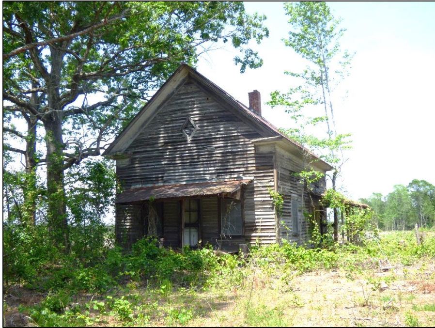
Photo 80: Peele's/Turkey Swamp School (MT0393), Northeast Oblique.
