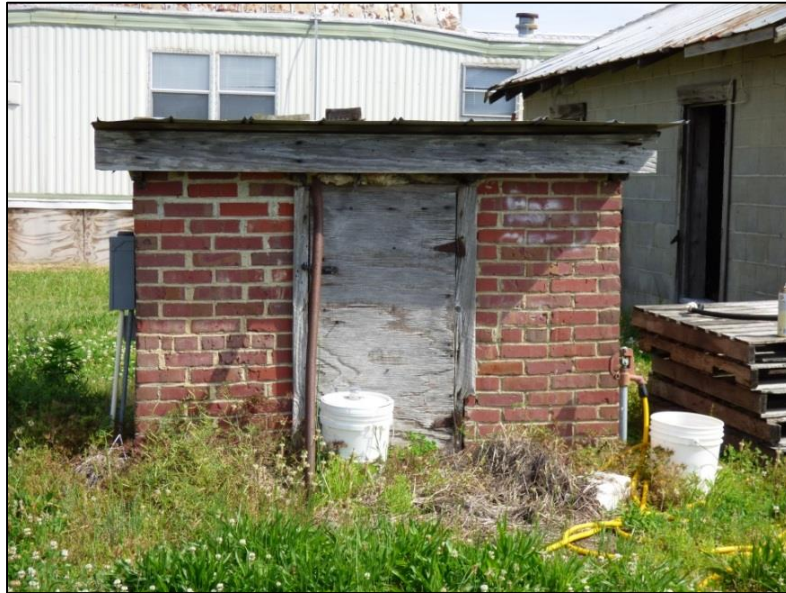
Photo 52: Pumphouse, South Elevation.
