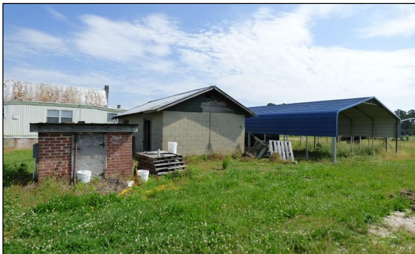
Photo 53: Pumphouse, Concrete-Block Outbuilding, and Carport, Looking Northeast.
