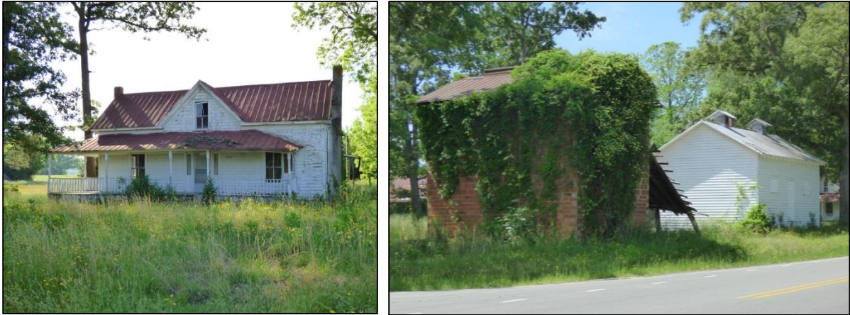
Photo 109: Dwelling (Left) and Associated Outbuildings (Right) of the Bowen Farm (MT0626)
