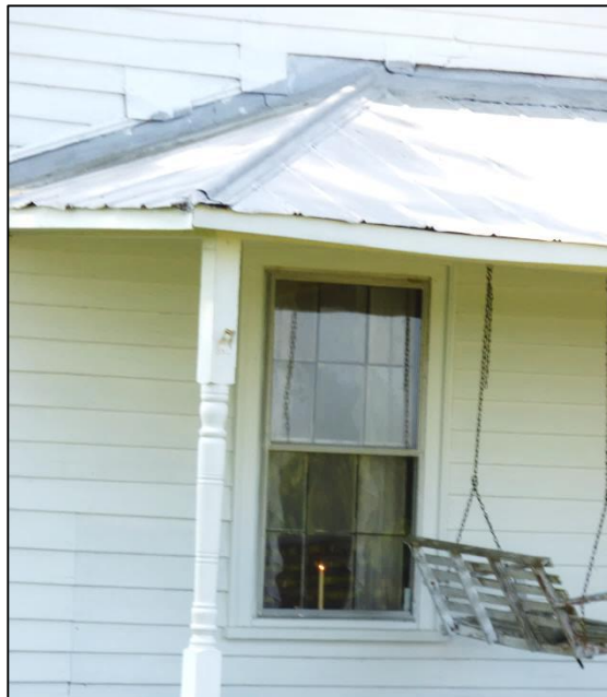
Photo 59: Dwelling, North Elevation Window Detail.
