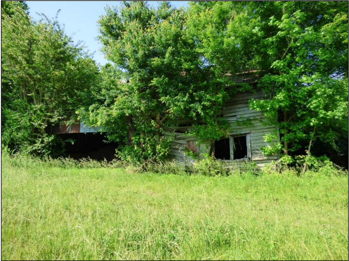
Photo 40: Possible Secondary Dwelling or Barn; Northeast Elevation.
