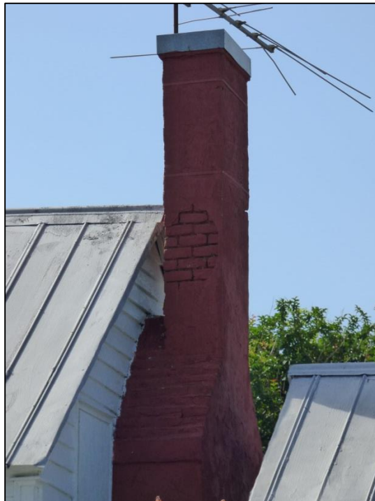
Photo 58: Dwelling, West Elevation Chimney Detail.
