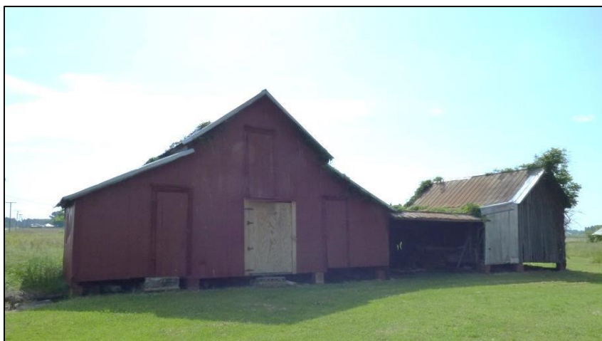
Photo 68: Packhouse (Left), Machine Shed (Middle), and Corn Barn (Right), Looking Southeast.
