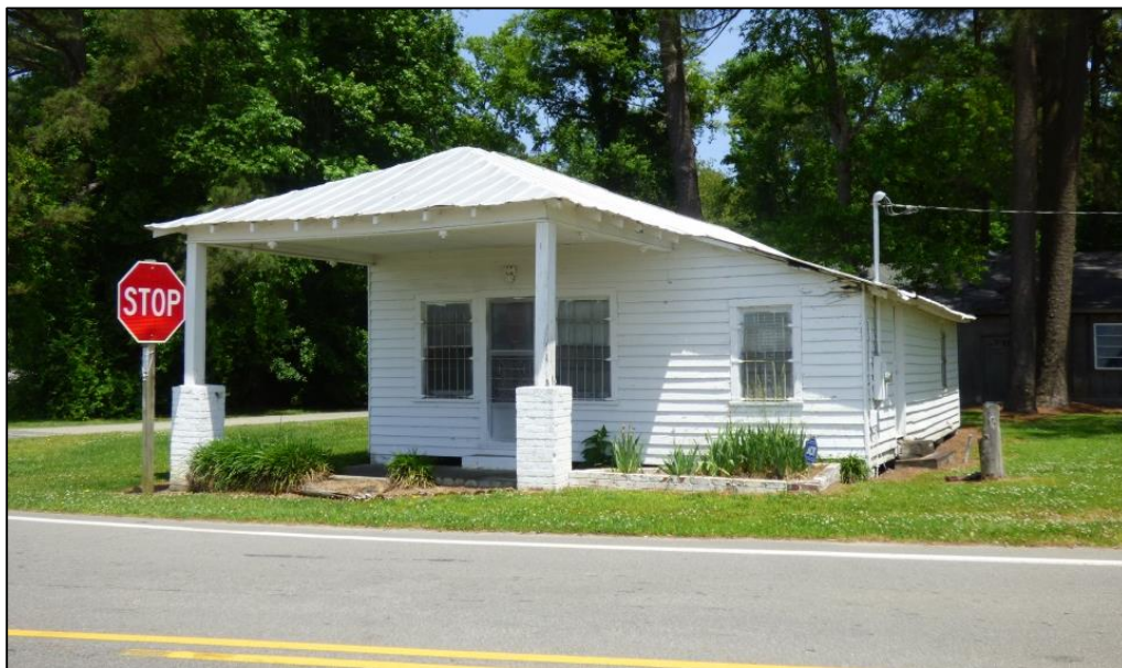
Photo 10: (Former) Fred McDaniels Store (MT0397) at the Intersection of Ed's Grocery Road (SR1106) and Everetts Road (SR 1138).
