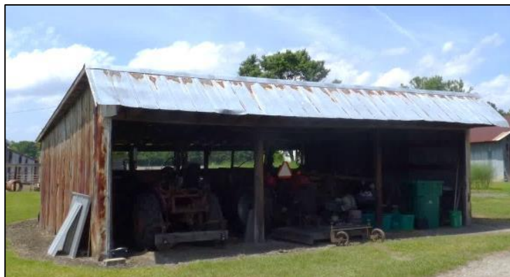
Photo 103: Southwest Oblique of the Garage/Machine Shed.
