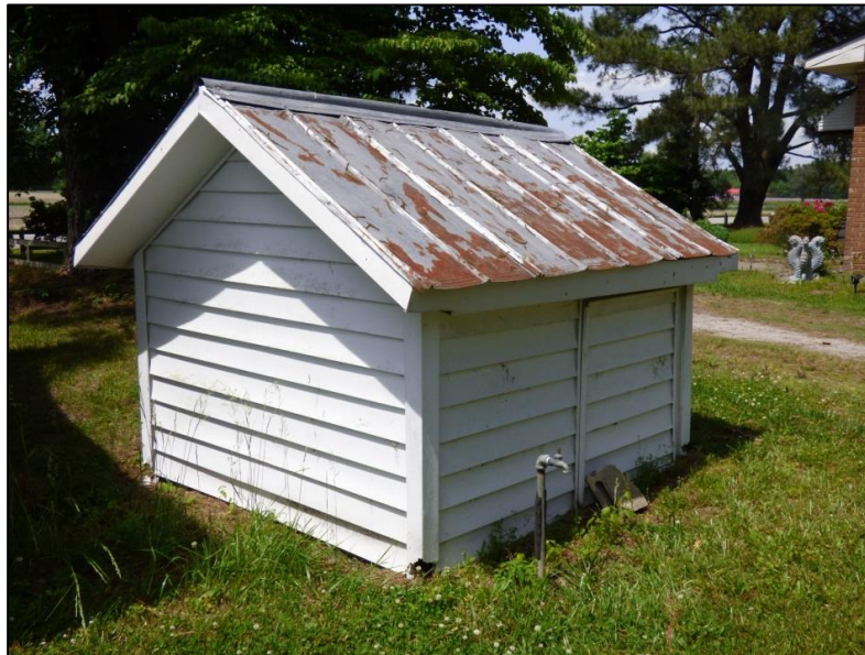
Photo 116: Pumphouse, South Oblique.
