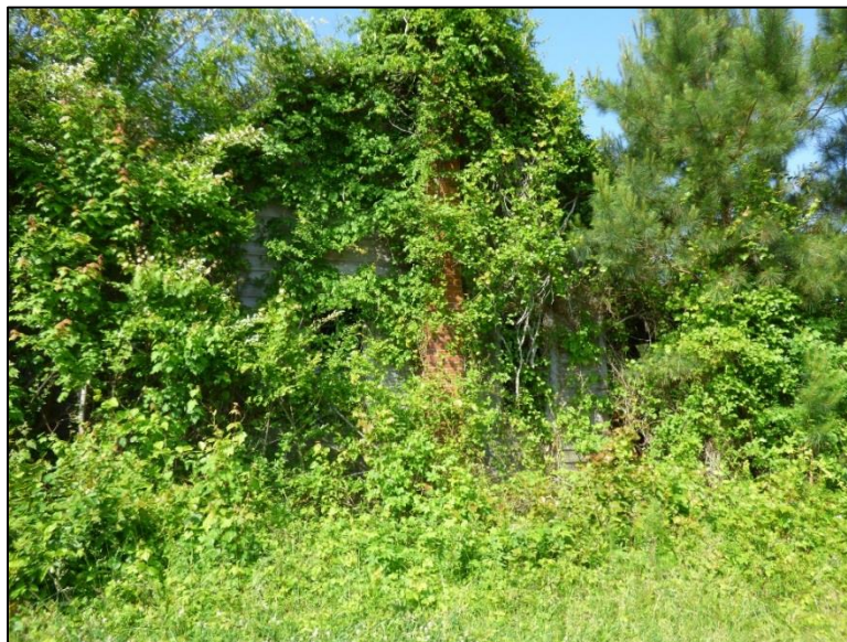
Photo 37: Tenant House, Northeast Elevation.
