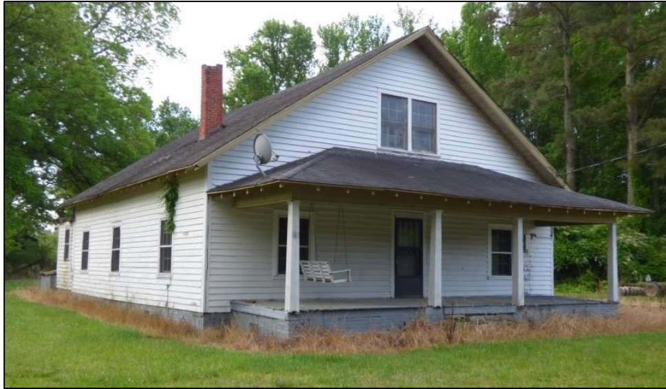
Photo 121: C.M. Wynn House, Northeast Oblique.
