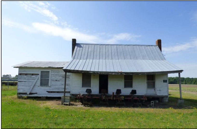
Photo 117: Façade (North Elevation) of the Alexander Mobley House.
