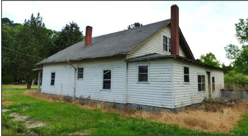
Photo 125: C.M. Wynn House, Southwest Oblique.
