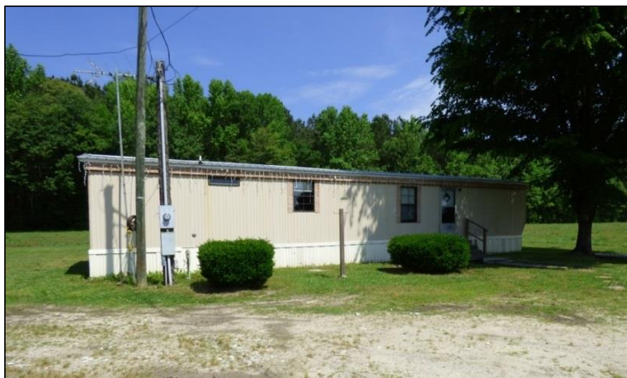
Photo 6: Mobile Home, Southeast Elevation.
