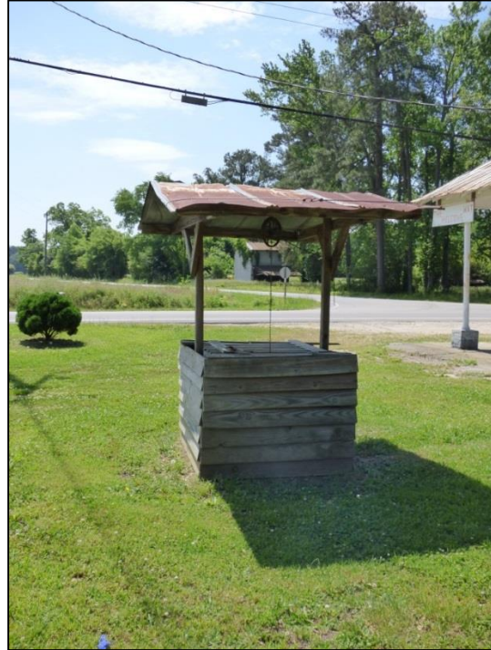
Photo 7: Well House, Looking South.
