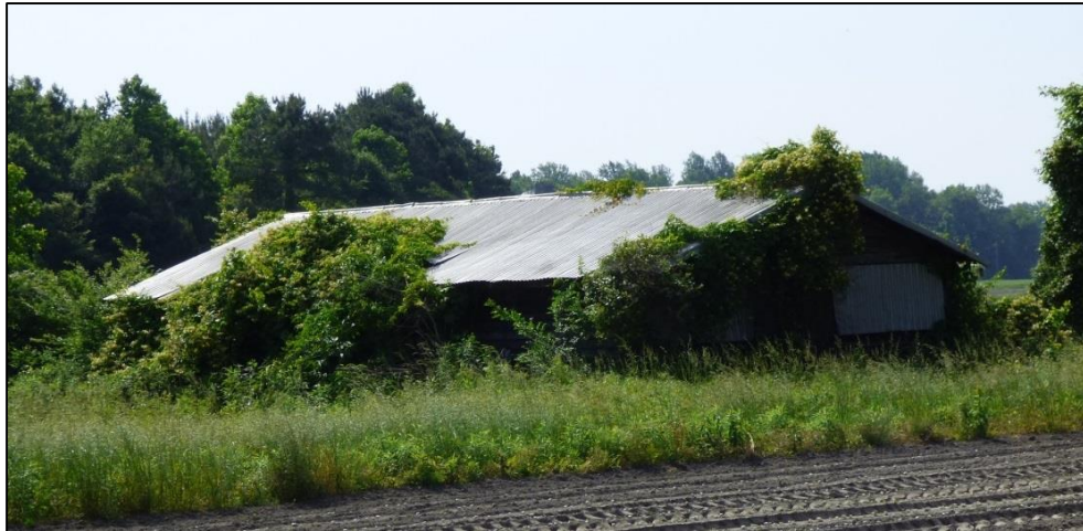
Photo 71: Hog Parlor, Northwest Oblique.
